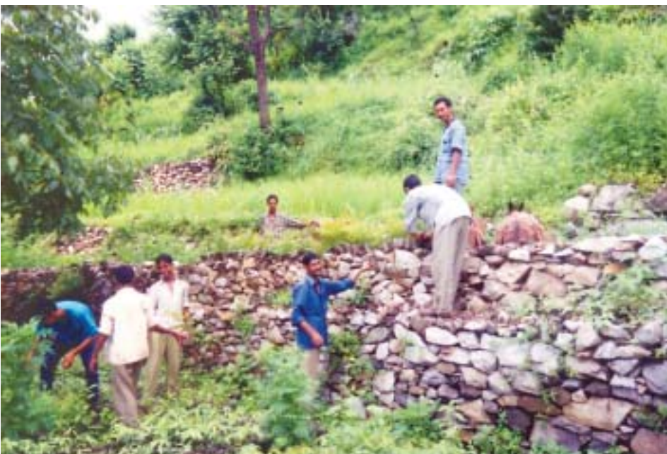
(Clockwise from top left) Trenches ready for water retention and plantation, saplings of different species of plants outside one of the several nurseries set up in the watershed area just before transportation, and construction of a bund in progress
